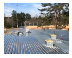
Figure 2 S. Atl – Mechanical Roof Curbs
